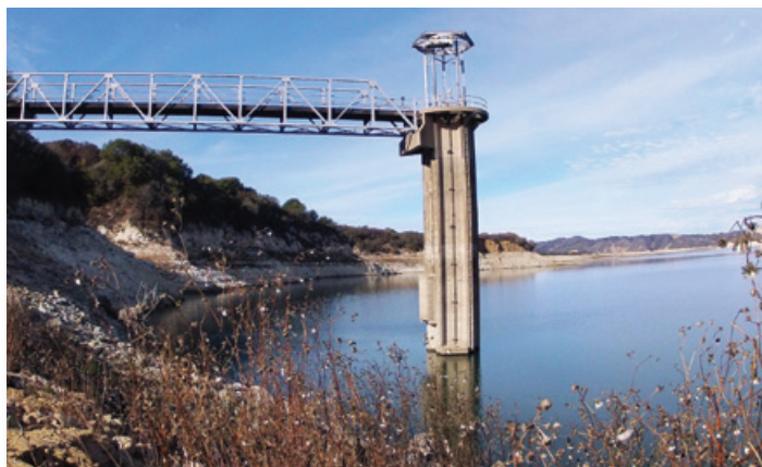
The COMB Emergency Pumping System at Lake Cachuma will ensure water deliveries even as lake levels fall.
