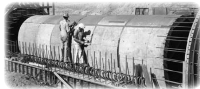
Working on a portion of the Cachuma project.
